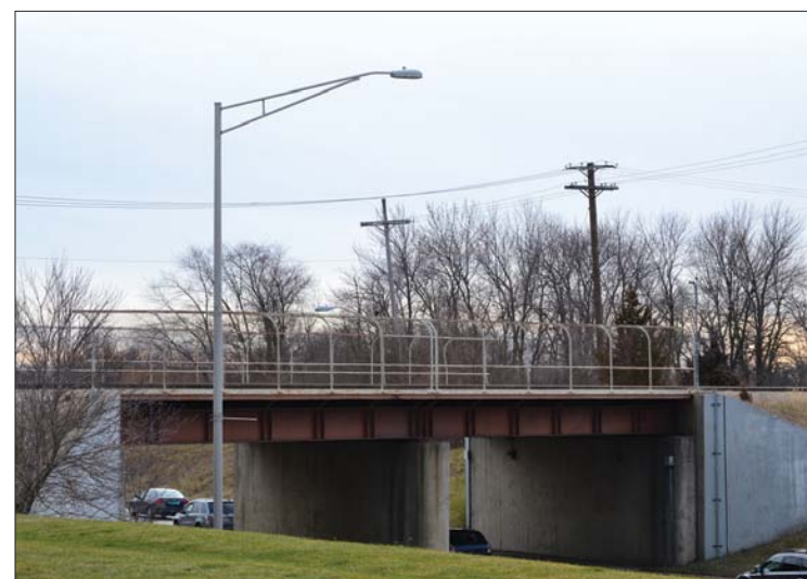
Figure 3.18 IFC railroad overpass at Harlem Ave.
