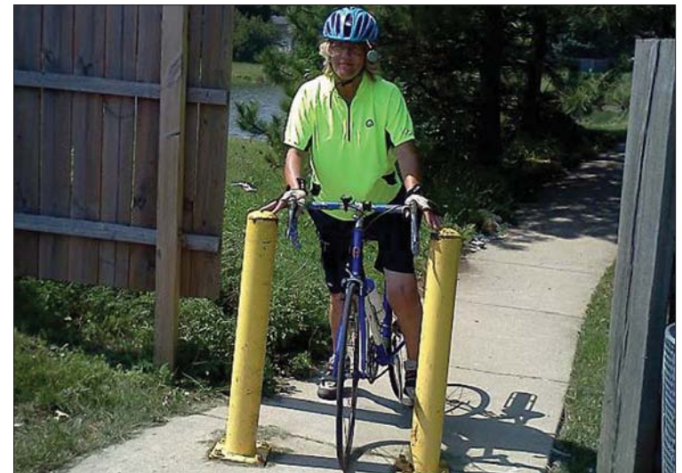
Figure 3.22 Example of bollards as pedestrian barriers
