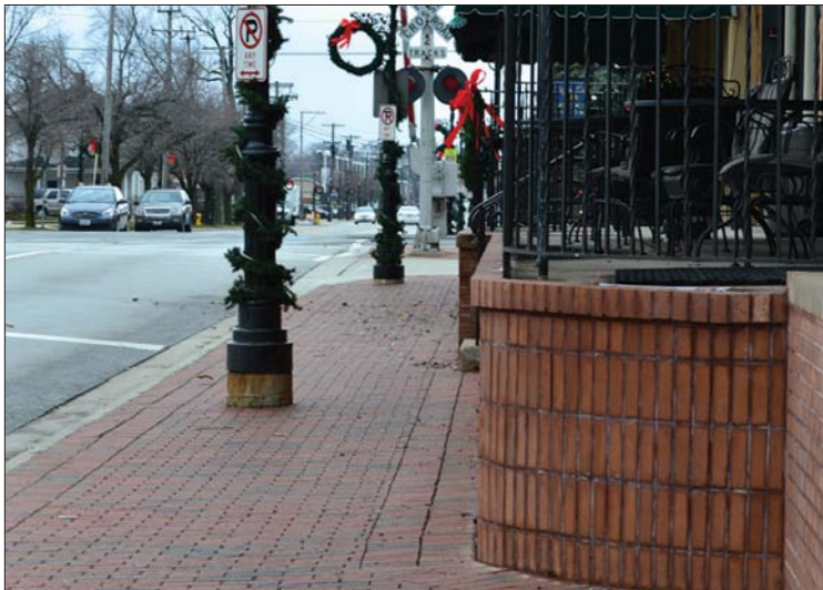
Figure 3.3 A narrow sidewalk along Oak Park Ave.
